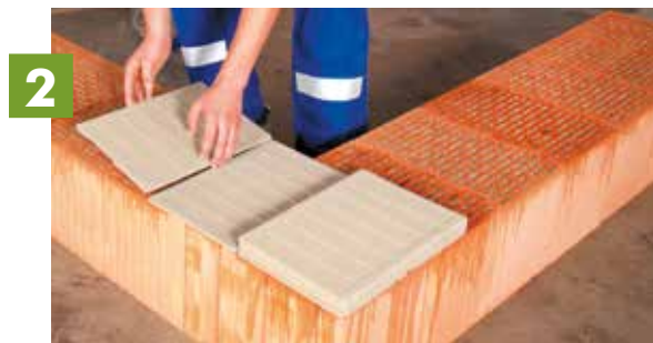
Lay on maxit mörtelpads
