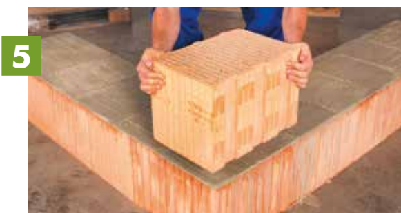
Position brick with full surface
