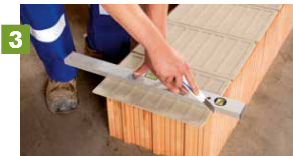
Cut to size if necessary
