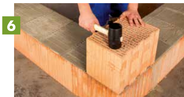
Align brick in usual way
